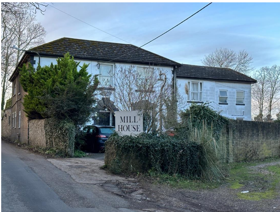
Mill House: The property is side-on to the road.
